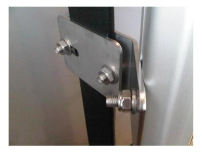
The side mounting brackets are used to attach the VR to the upright rail instead of the rungs to maximize the tread area on narrow ladders which could create a climbing hazard if the vertical rail was secured to the centre of the rungs, or to the side.
