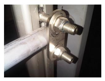
This Rung Mounting kit is to be used when securing the Vertical Rail to a steel ladder which has horizontal rungs; it can be fitted to the middle or the side, as shown. These are to be fitted between 0.5 m & 1 m from the end of each individual section.
