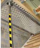
Safety Note:The mat is not suitable to be loaded out with materials. Maximum spread load is 150kg
