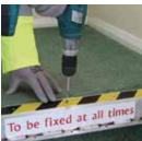
Safety Note: The frame must be secured on the top riser with at least 2 x 38 mm screws.
