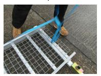
Tie the supplied strap to the top rung of the Board-Walk.
