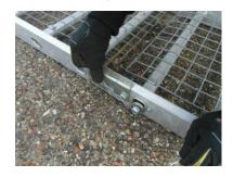
When the Locking pin is in place secure with the supplied 'R' clip.
