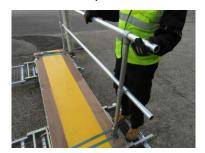
Fit the top rail and secure both the mid and top rails to the end uprights with the grub screws provided.
