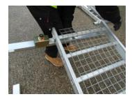
Attach the first support Batten to the Board-Walk section using the captivated pins in the hole in the stiles.
