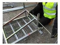
Remove the height adjusting pin and raise the height of the platform to the horizontal position. Remember this is usually set at Roof level.
