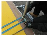
Fit the two end uprights into the sockets and secure with the supplied pin and 'R' clip.
