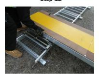
Position the Cat-Walk onto the trolleys.
