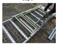
Install the two number trolleys on the separate tracks of Board-Walk. Positioning the rollers on the stiles of the staging and engaging the hooks on a rung.
