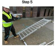
With the strap tied on securely lower the Board-Walk panel onto the roof. You would repeat these steps for additional Board-Walk panels. This picture is for demonstration purposes only.
