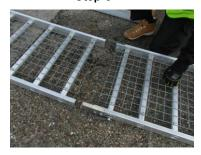
Connecting Additional Board-Walk together, follow STEP 4 & 5 in these instructions for laying the board walk into position.
